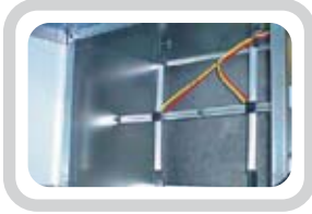
air flow sensor
